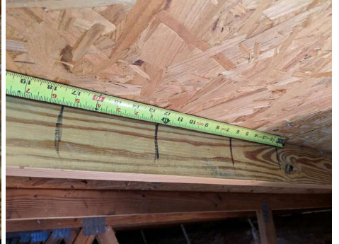
ROOF DECK ATTACHMENT SPACING
