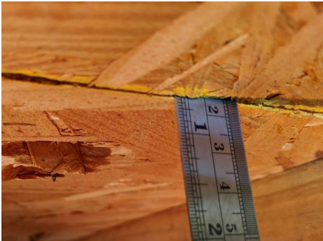
ROOF DECK THICKNESS
