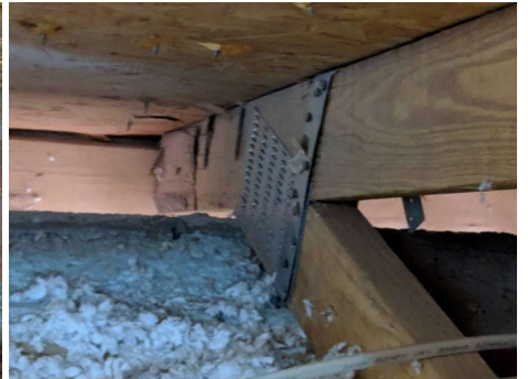
ROOF TO WALL ATTACHMENT
