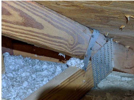
ROOF TO WALL ATTACHMENT
